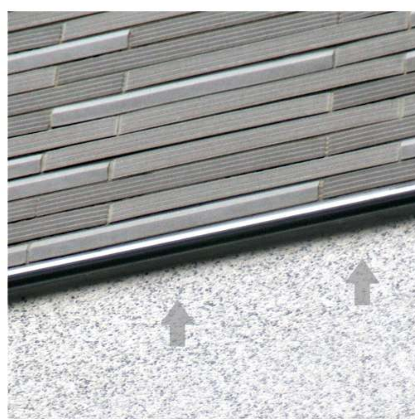
Construction Site Photo
