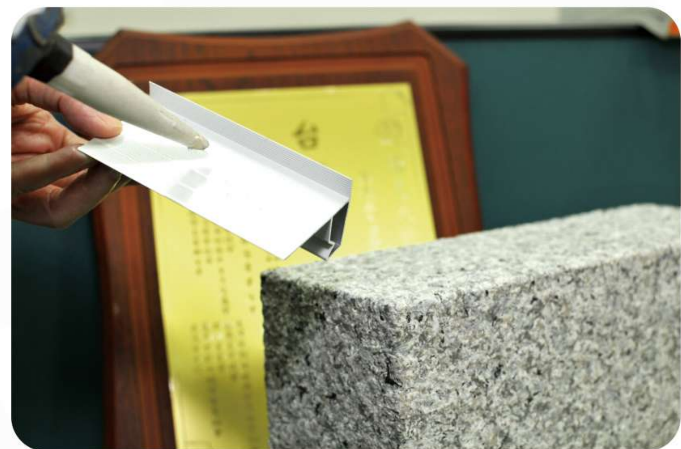
02 Apply silicone sealant to the back of the water drip edge.
