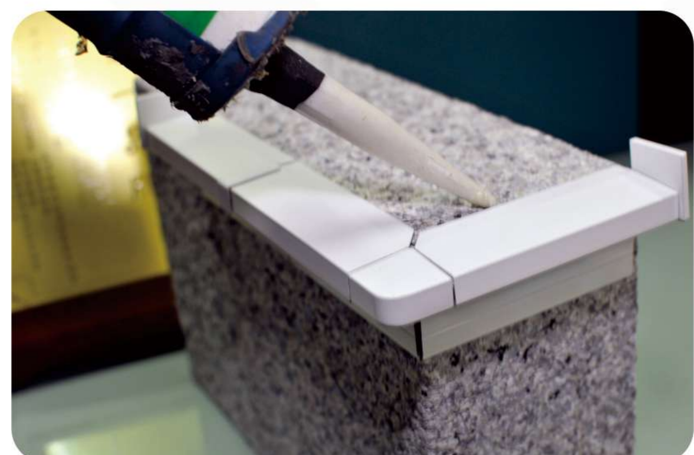
06 Apply silicone sealant along the seams.
